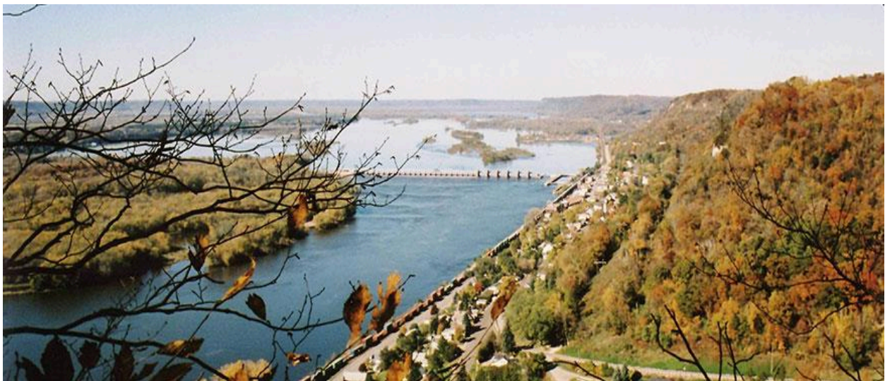
Lock and Dam No. 4 in Alma, WI. Photo courtesy of Buffalo County.
